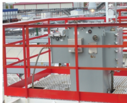
Explosion-proof flexible high-voltage bushing assembly of NWL OILPRC power unit
