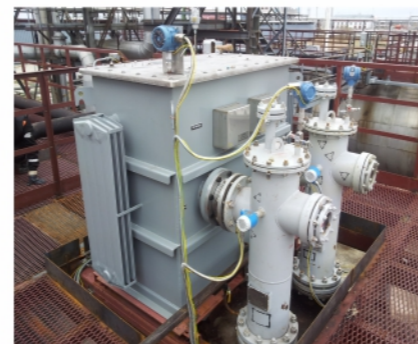
Explosion-proof oil-filled high-voltage bushing assembly of NWL OILPRC power unit
