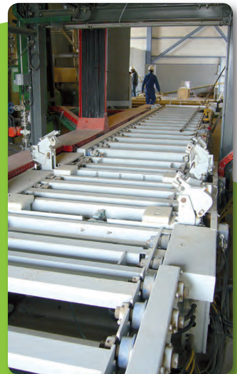
Fully automatic operated roller conveyor for casting molds
